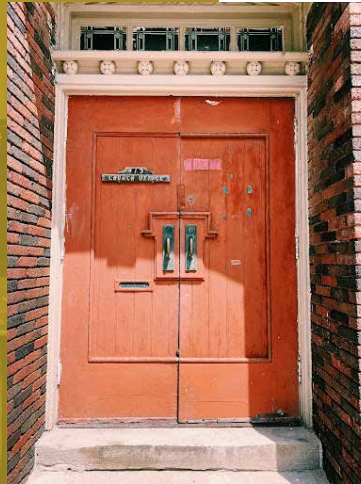
Front door detail
